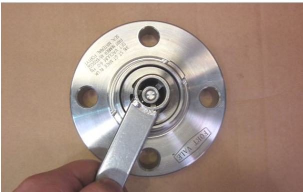
Step 9. Locate the locking tool in the spring pad.
